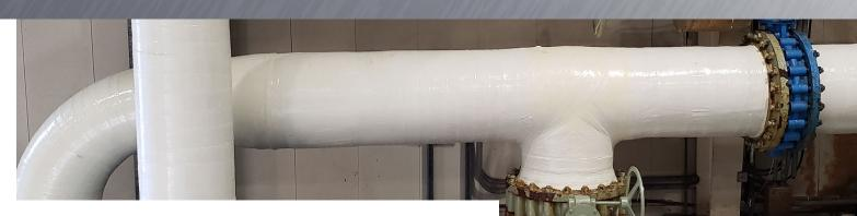
**DEACON<sup>®</sup> SEAL WRAP<sup>™</sup>** solutions are engineered to tackle pipe-related challenges. From fast and slow cure reinforcements to high-temperature resilience, our wateractivated fiberglass wrap system ensures your pipes, tanks, and pressure vessels are fortified, sealed, and maintained.
