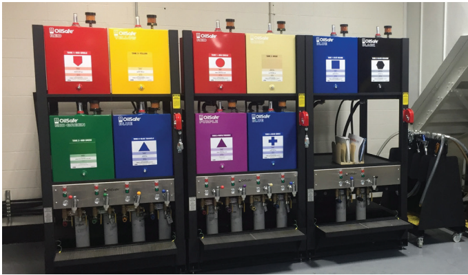
Figure 3: New lube room
