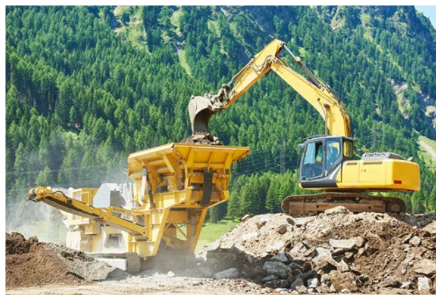
Figure 4. Crusher being fed by a large excavator.
