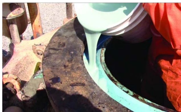
Figure 3. Deacon Crush-Bac being poured.
