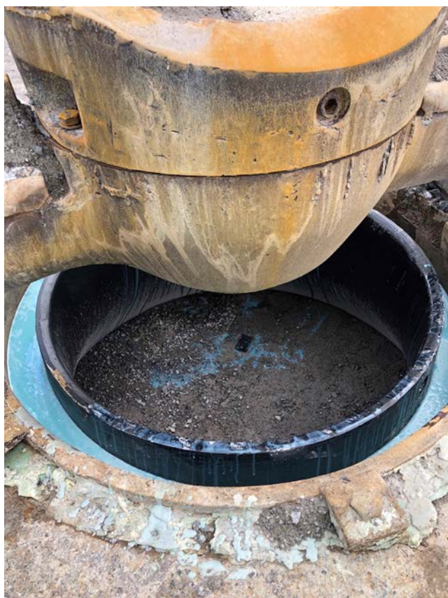
Figure 1. Deacon Crush-Bac backing compound (blue).
