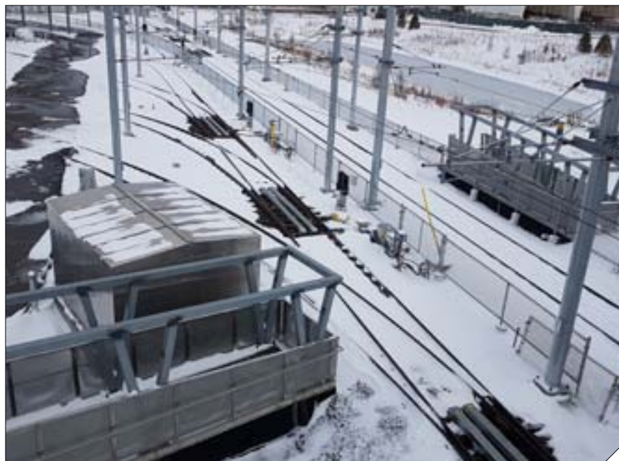
The Eglinton Crosstown LRT Maintenance and Service Facility in Toronto uses Thermon Fastrax Hellfire 400 gas-fired switch heaters, shown here installed and operational. 50 of these units are installed in the yard.
